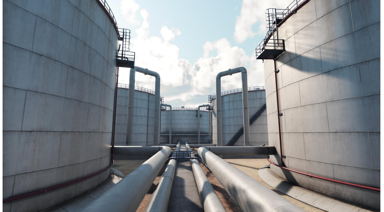
Pekerjaan Cleaning-Blowdown Oil Storage Tank
